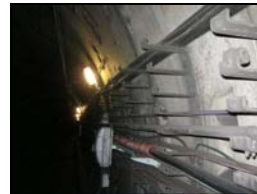
North Greenwich Site
