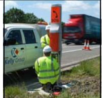
Installation of ERT
